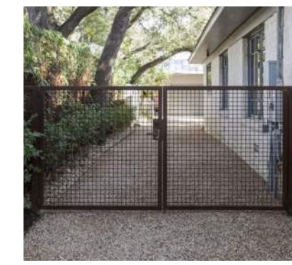
WELDED WIRE MESH FENCE
