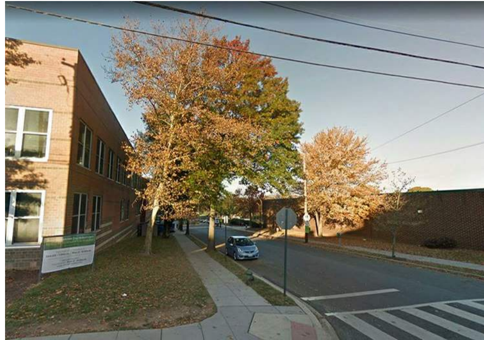
2. 42ND STREET LOOKING WEST
