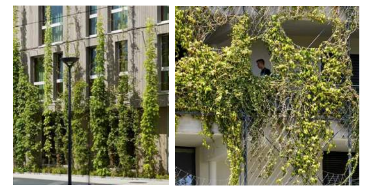
GREEN SCREEN: WIRE ROPE (LEFT), WIRE MESH (RIGHT)
