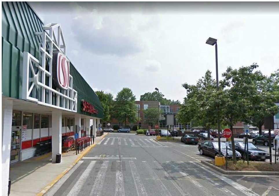
4. SAFEWAY BUILDING LOOKING SOUTH
